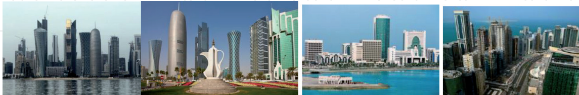
Figure 2. Contemporary architecture in Doha city.
