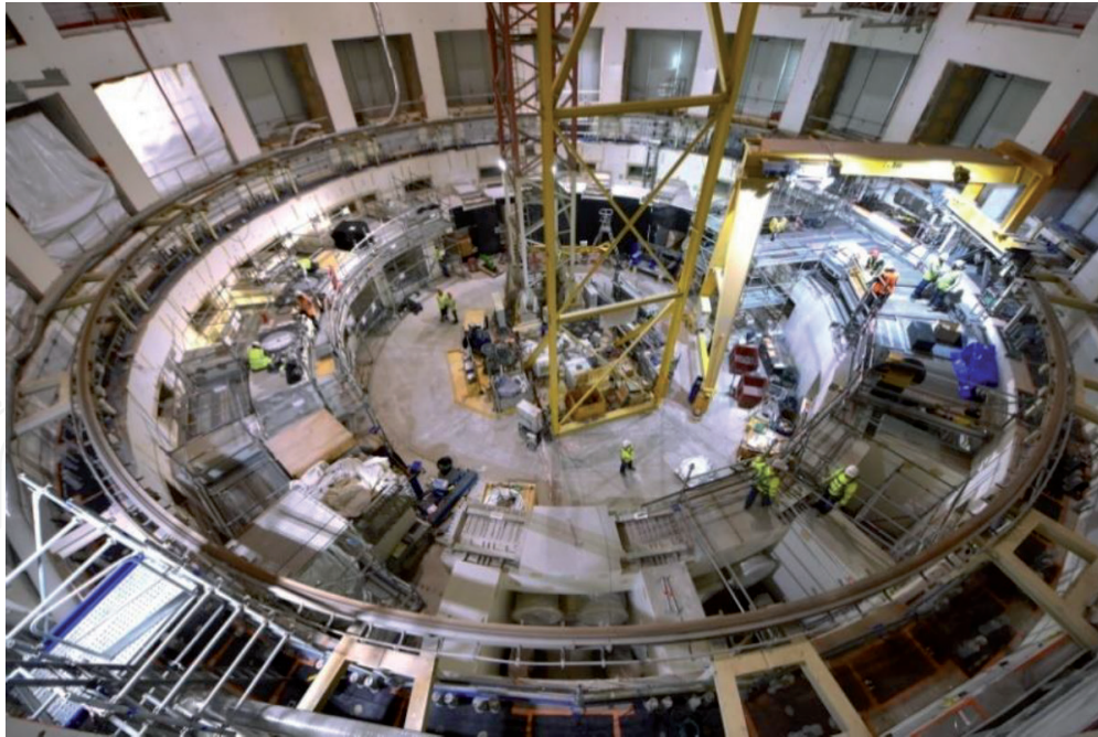
Figure 4. International thermonuclear experimental reactor ITER (ITER).
