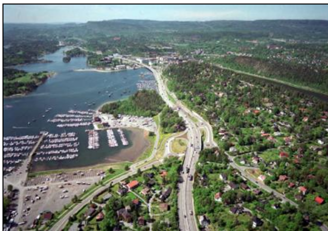
Figure B.11: E 18 west, photo from NPRA (2011).
