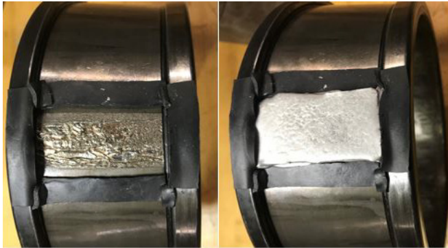
Figure 7. Casting procedure using Bismuth; spalled surface outlined with tacky tape (left); Bismuth alloy cast (right)
