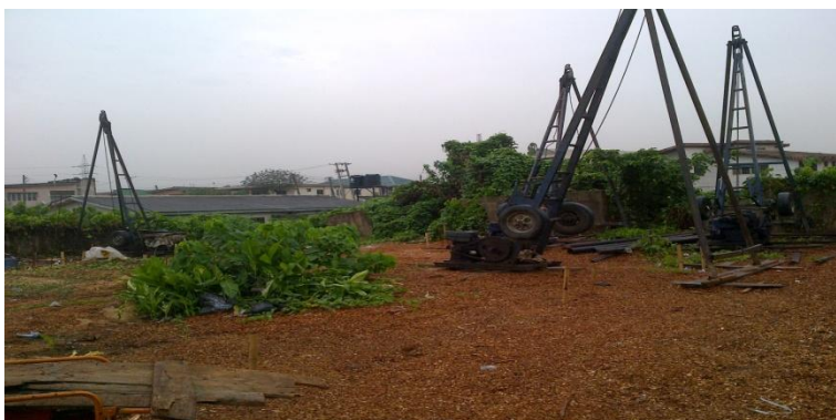
Figure 3: Pile driving machines in place
