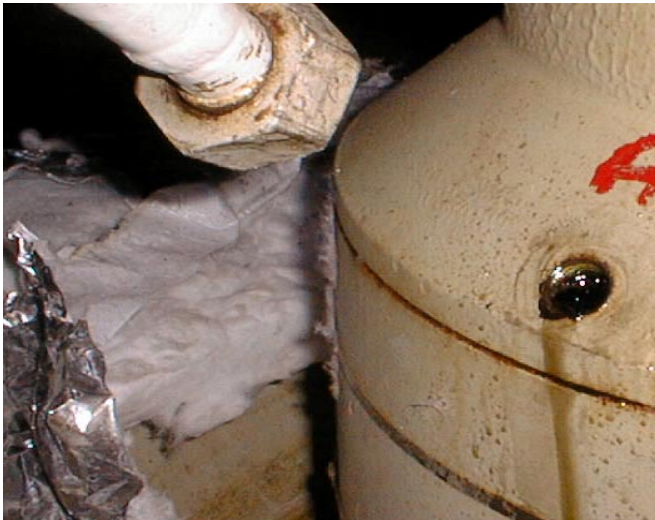
Picture 5. Annulus liquid out of the vent port
