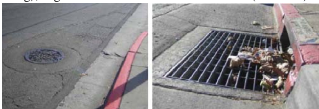
Fig. 10 Manhole and Storm Drain in front of Station #1
