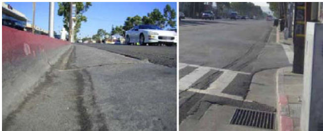
Fig. 9 Left: road Crown right before Station #2 (4.75-4.15 deg); Right: Road Crown from the Crossroad (144 Ave.)
