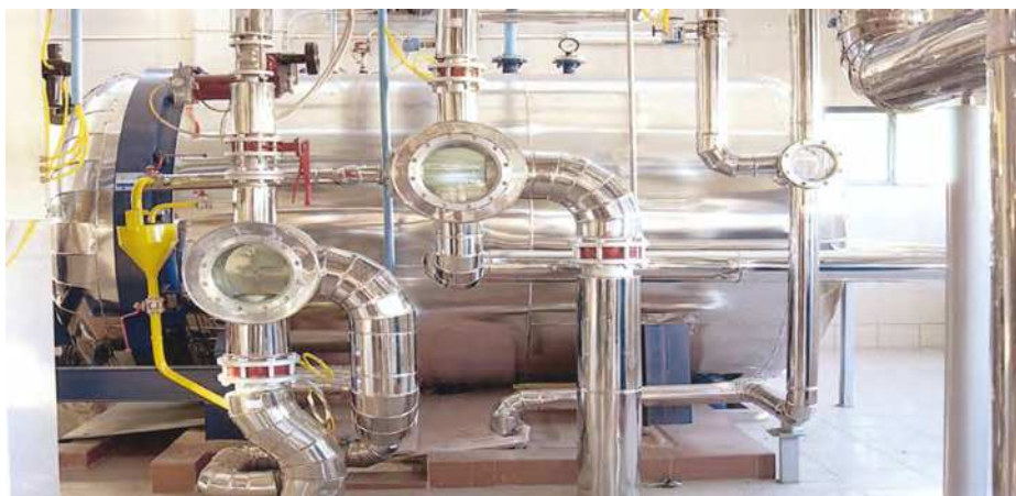
Fig. 9. Winterization filters
