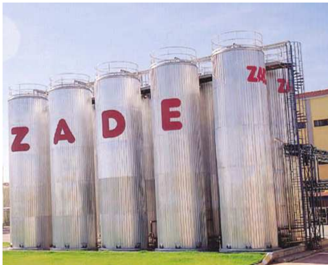
Fig. 11. Refined Oil Silos
