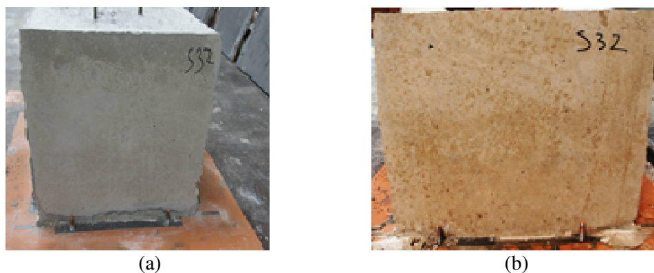
Fig. 2 : Concrete facing: (a) with a new wall; (b) with used wall
