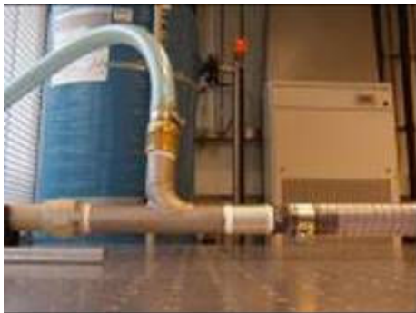
Figure 1: Water-air mixing point.
