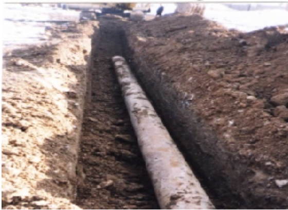
Fig. 8: Installed pipe in conduit
