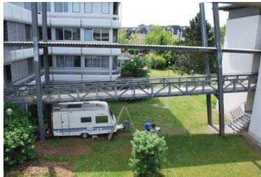
Fig. 13. North view of the bridge subjected to monitoring.
