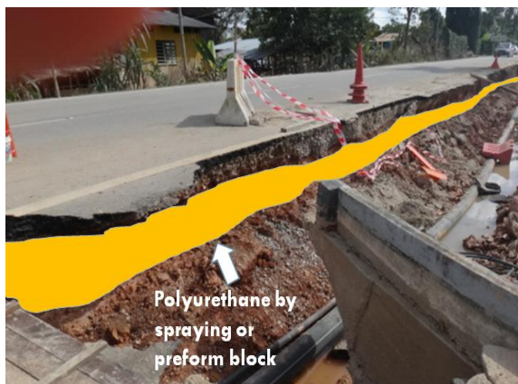
Fig. 1: Polyurethane layer by spraying or preformed block
