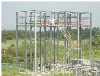
Fig. 4. Outdoor exposure test facility
