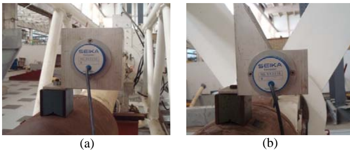
Figure 9 – Inclinometers (a) 01 and (b) 02
