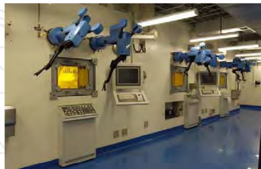
Figure 2. INVAP Mo-99 Production Facility at the OPAL Reactor
