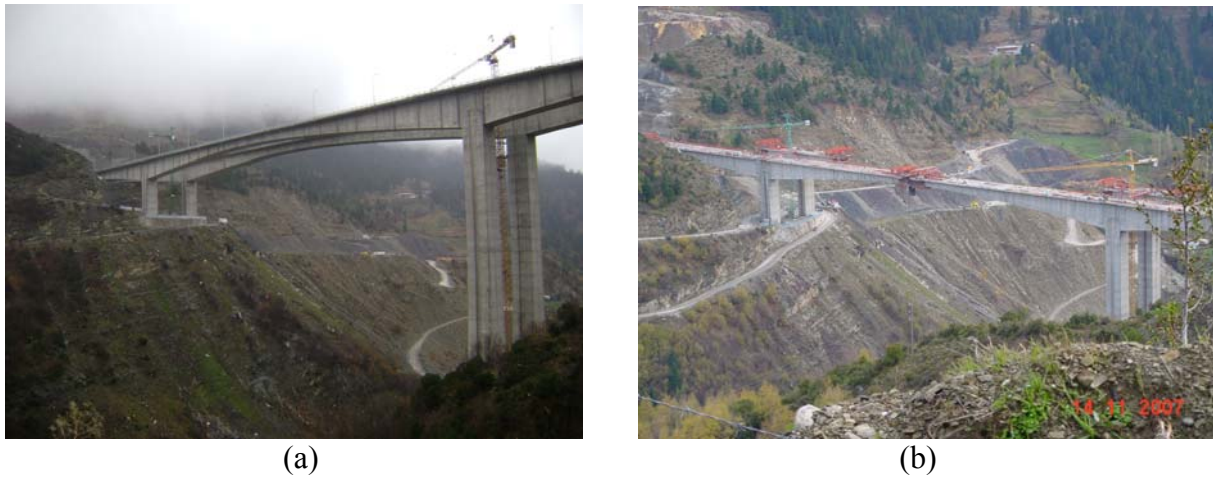
Figure 2: Metsovo bridge, (a) General view, (b) key of central span.
