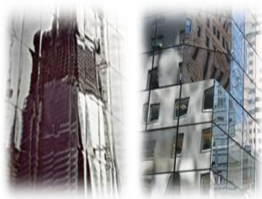
Fig. 3 (A) and (B) Shows the Reflection and Distortion on the Surface of Building
