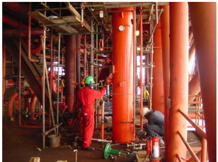
Figure 4 – Installation of replacement fuel gas scrubber during offshore TAR.
