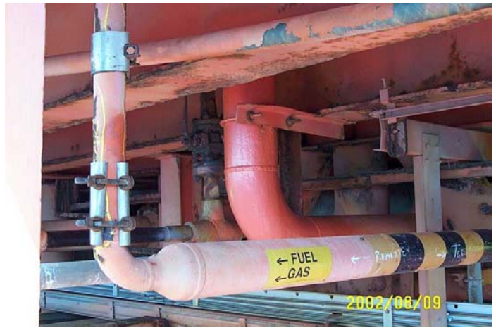
Figure 3 – Temporarily repaired fuel gas line replaced during offshore TAR.
