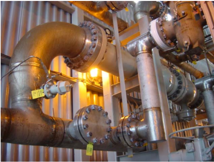
Figure 10 – Duplex stainless steel flowlines and production manifold on the Kapok platform.
