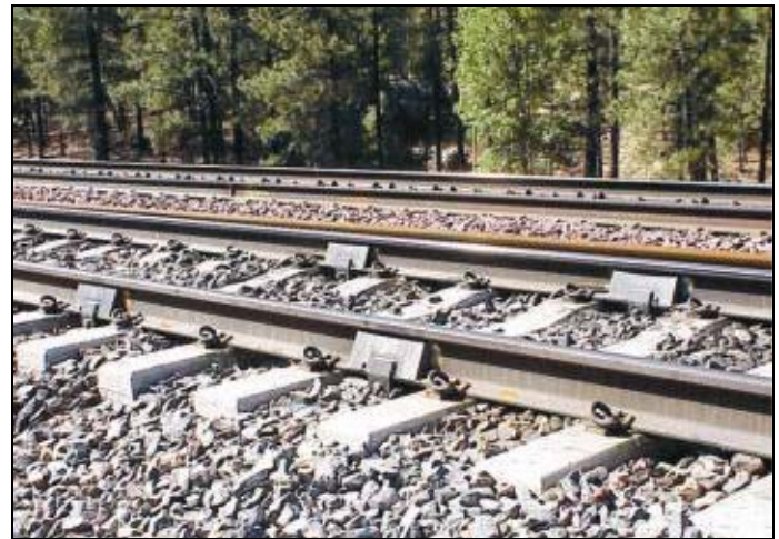
Figure 5. TPD Strain Gage Installation
