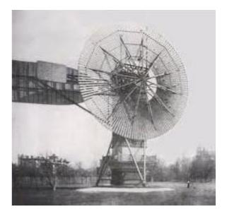
Figure 3 Charles F. Brush's wind turbine (1887, Cleveland, Ohio), the world's first automatically operating wind turbine for electricity generation.
