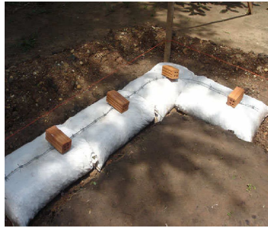
Figure-2- Earthbag Construction
