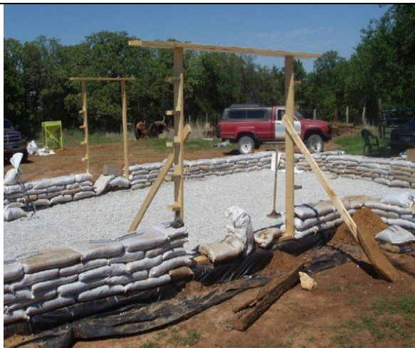
Figure-3- Earthbag Construction
