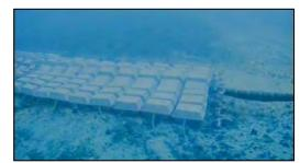
Figure 4 – Mattress over a pipeline
