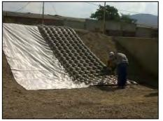
Figure 2 - Mattress placement on slopes
