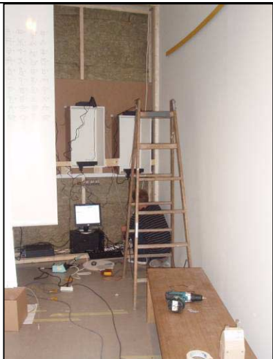
(a) Building the three listening posts. Loudspeakers, lights and a wall sheet with text are installed in each box behind the holes.
