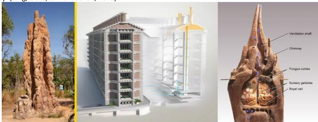
Figure 9 The Eastgate Center and termite nest section plan (Source National Geographic)
