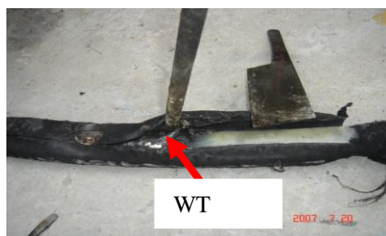
Figure 2.白 35 fault caused by the water tree
