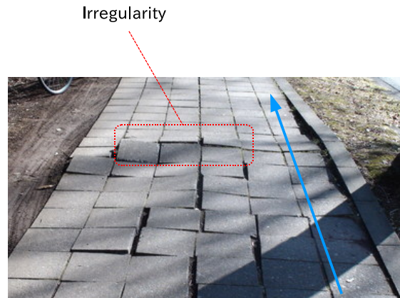
Fig. 8. Experiment Environment (C): This sidewalk is bumpy, and has smooth irregularity.
