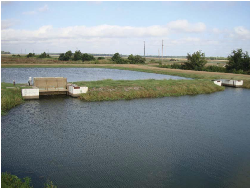
Figure 1.3 Split-pond system with slow rotating paddle wheel to provide water movement between the fish holding basin and the algal basin (Brown and Tucker 2013).
