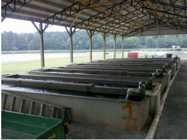
Figure 1.1 Flow through recirculating aquaculture system (RAS) at Auburn University.
