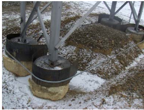
Figure 11. Four separate foundations tied.
