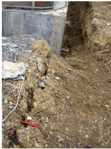
Figure 13. Reinforcement of footing of a masonry room.
