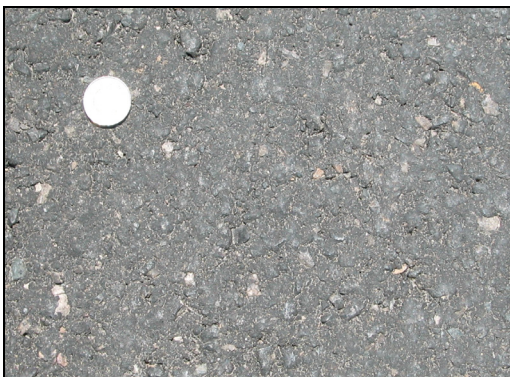
Figure 4. a) Finished Surface of CIR Mix
