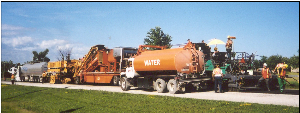
Figure 3. Cold-In-Place Recycled Expanded Asphalt Mix Train
