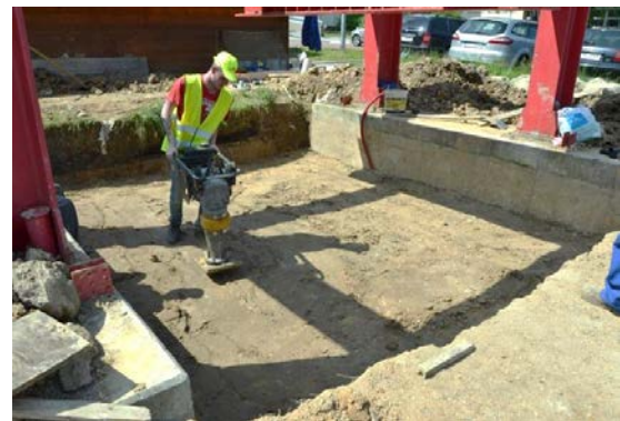
Fig. 3 Completion of sub-layers by compaction
