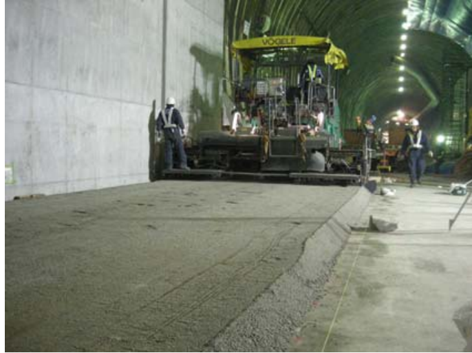
Figure 5. Spreading by Asphalt Finisher
