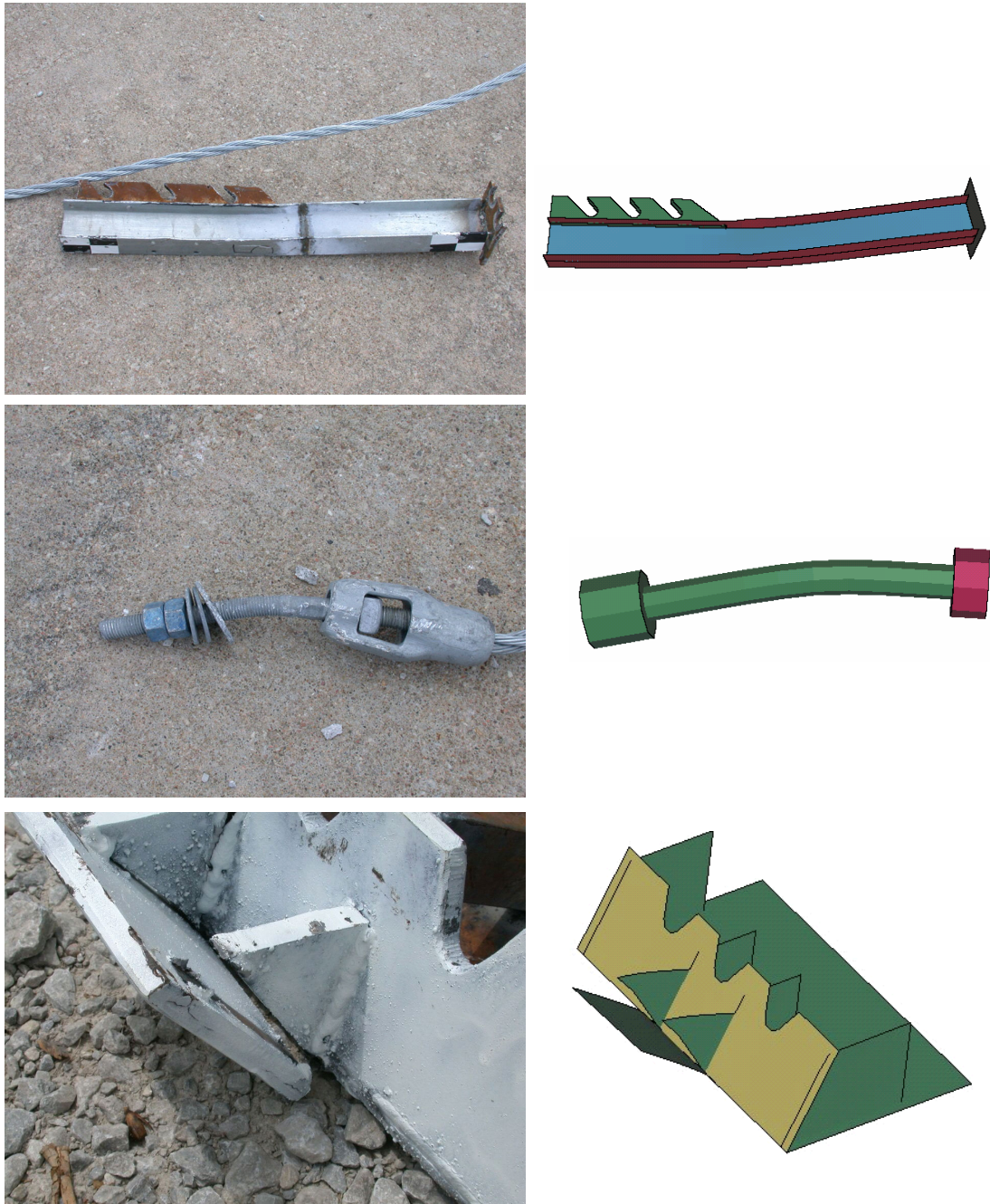
Figure 7. Deformation Comparison - Post, Cable End Fitting, and Anchor Bracket
