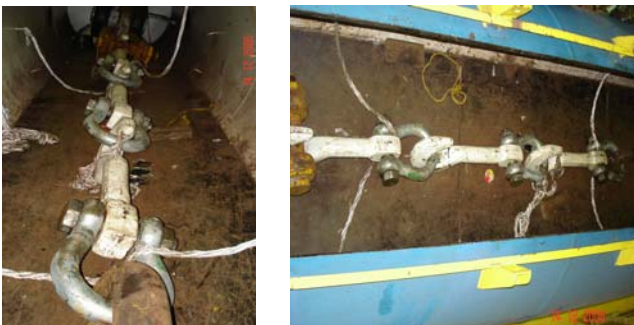
Figures 10 and 11 – KS12 Hook with and shackles and chain links connection Details
