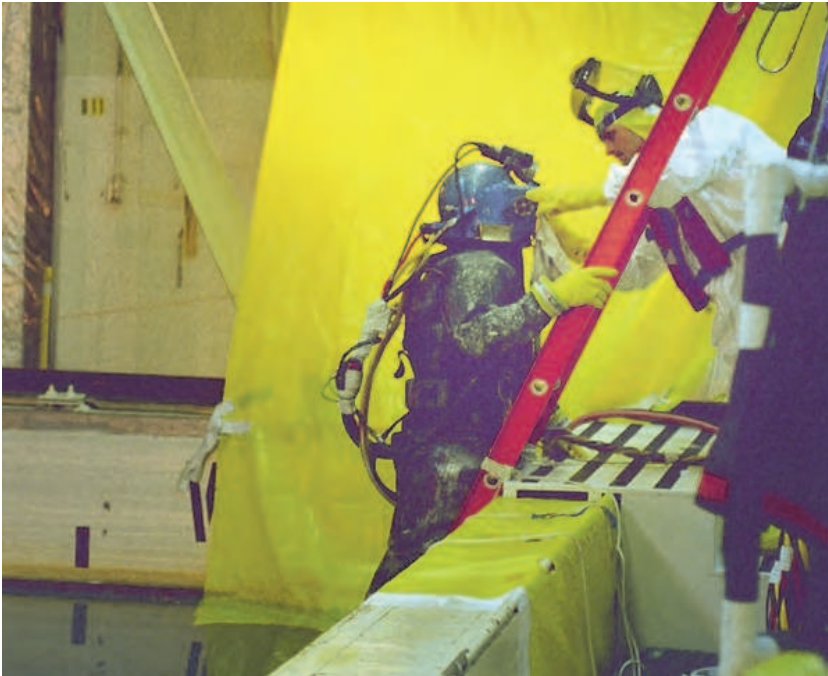
Fig. 1. Diver at INL completing entry into basin for underwater cleaning and coating.
