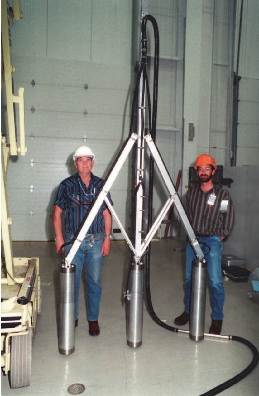
Fig. 3. Multi Detector Basin Scanning Array for INTEC-603.
