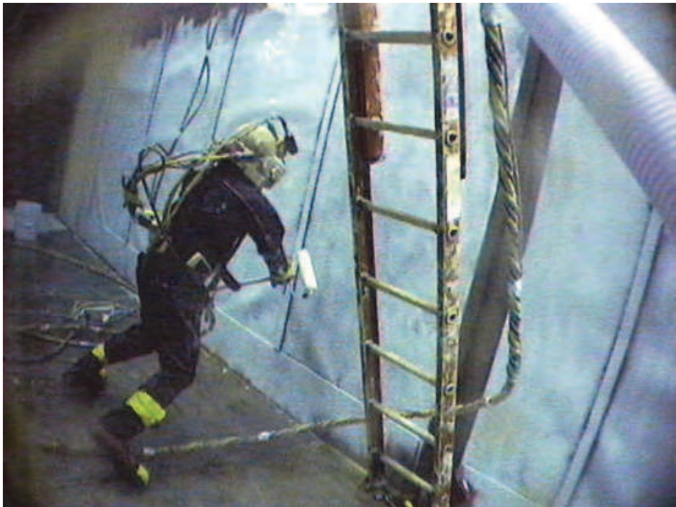
Fig. 2. Special two hose roller system used for wall coating at the MTR pool.
