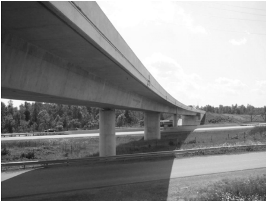
Photo Courtesy of Boschung America, LLC
