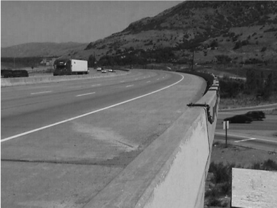
Photo courtesy of Boschung America, LLC
