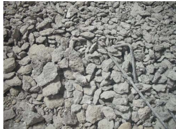
Figure 1. Demolished walls and piles
