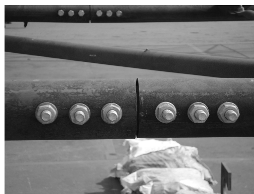
Fig.2. Tube sleeve connection
