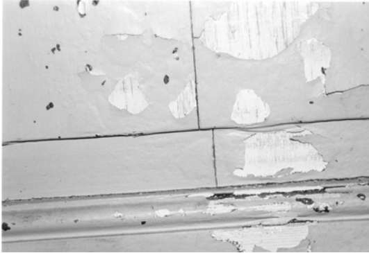
Figure 6. Flaking off lacquer
