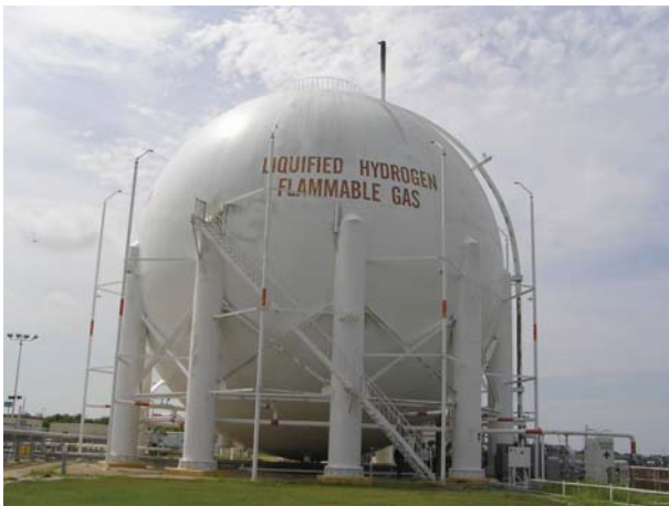
Figure 1. Liquid Hydrogen Storage Tank at Launch Complex 39, Kennedy Space Center
