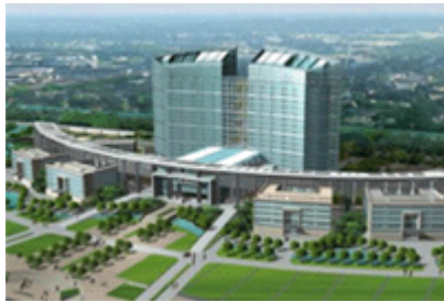
Fig. 1. Front view of the project
