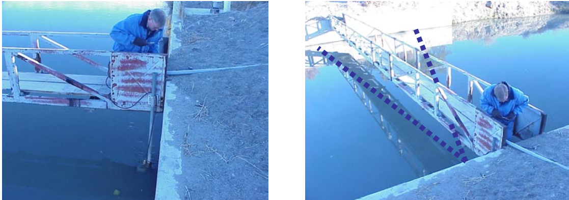
Figure 4. SonTek/YSI Argonaut SL installed in a canal
