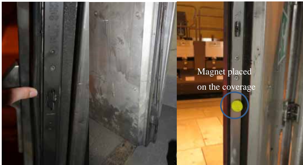
Figure 6: From left to right: contaminated locking pin, brake dust behind the coverage, magnet placed on coverage [5]
