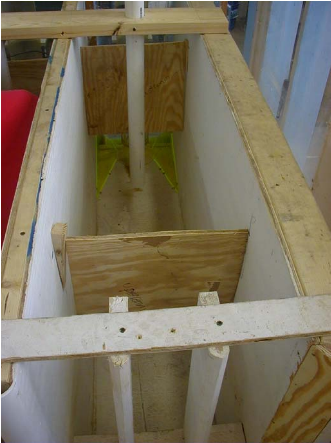
Photo 8 Curtain Walls, Piers and Fillets & Splitters
