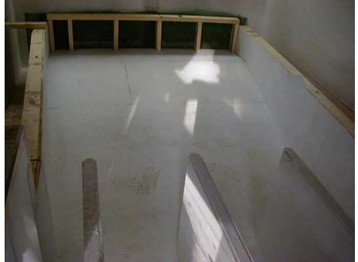
Photo 3 Sloping Ramp Transition
