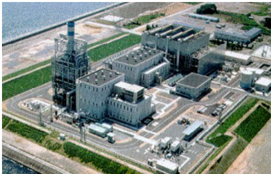
Figure 2. MHI in-house verification combined cycle power station, T-Point
