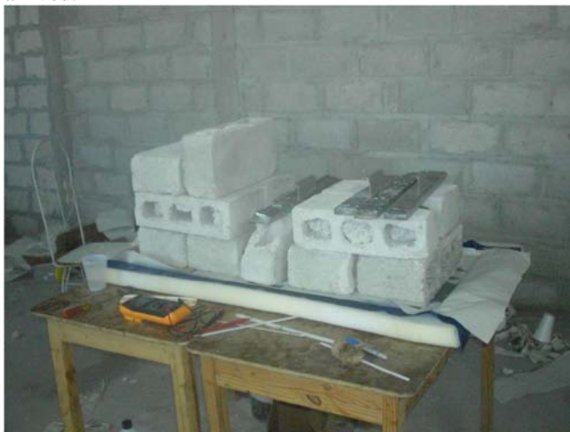
Fig 5 Low-tech laminating system using heavy weights, developed by Enersa in Haiti.
