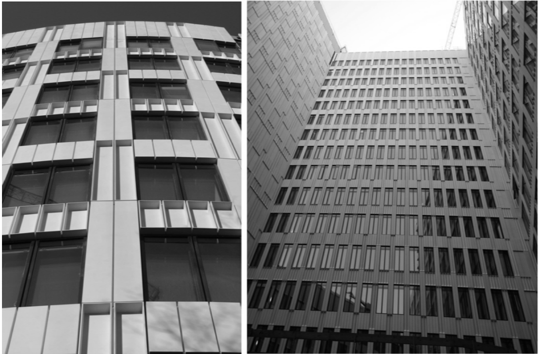
Figure. 5: Mounted Façade Elements on the Multistory Building “Leo”
