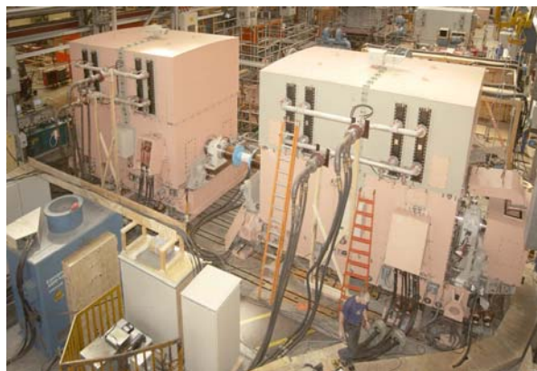
Fig4: Back-to-back performance test of two 65MW compressor driver motors in the Berlin motor plant. (The associated „drives“ are located outside the building)
