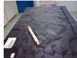
Fig.9. Visible delamination of the VIP fire protection fleece after temperature ageing at 80°C for about 1 month.
