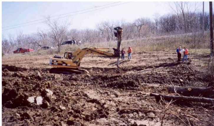
Figure 8 Construction for landslide repair, Dallas County
